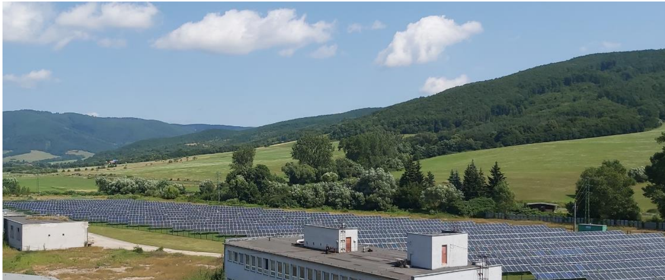
View of the photovoltaic plant in Lovinobaňa
